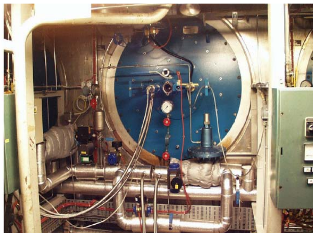
Burners for firing Pine oil a waste product for the paper industry
